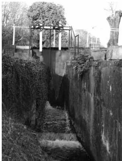
The mill race at Tetstill, where the Neen Sollars hydro electric generator will be installed.
